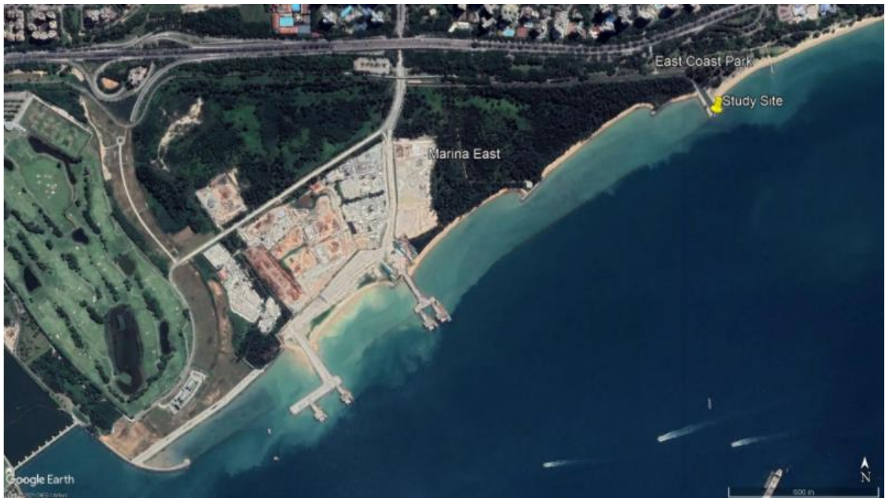
Fig. 2. Satellite map of the study site. The faint dark line parallel to shore is the rock bund. (Map: Google Earth. Image©CNES / Airbus. 29 June 2016).
