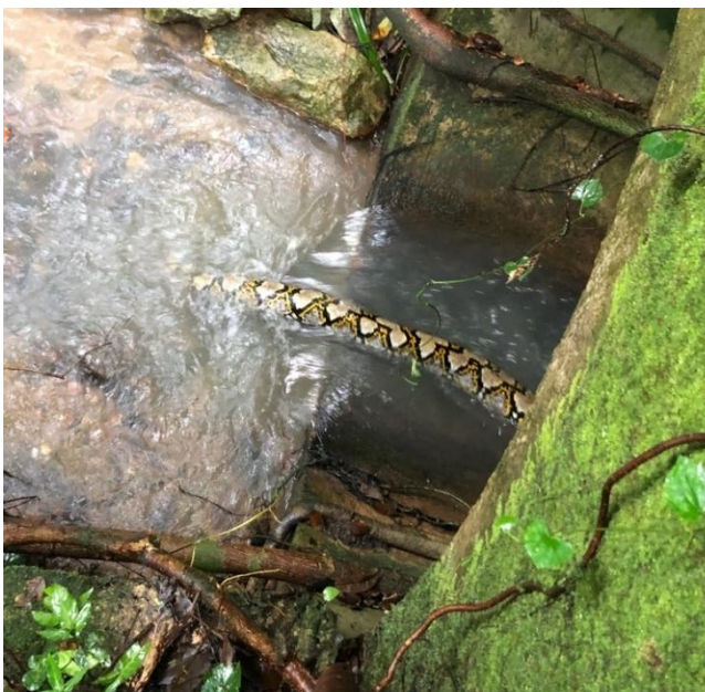
Fig. 1. The rear section of the snake as viewed from above the culvert. (Photograph by: Serene H. Y. See).
