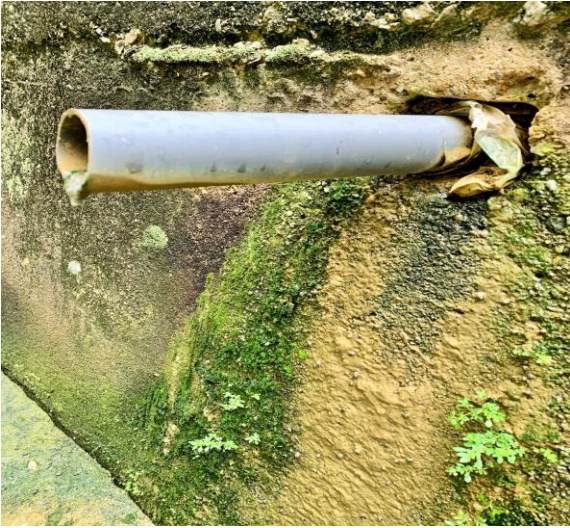
Fig. 1. Weep hole on a concrete wall.
