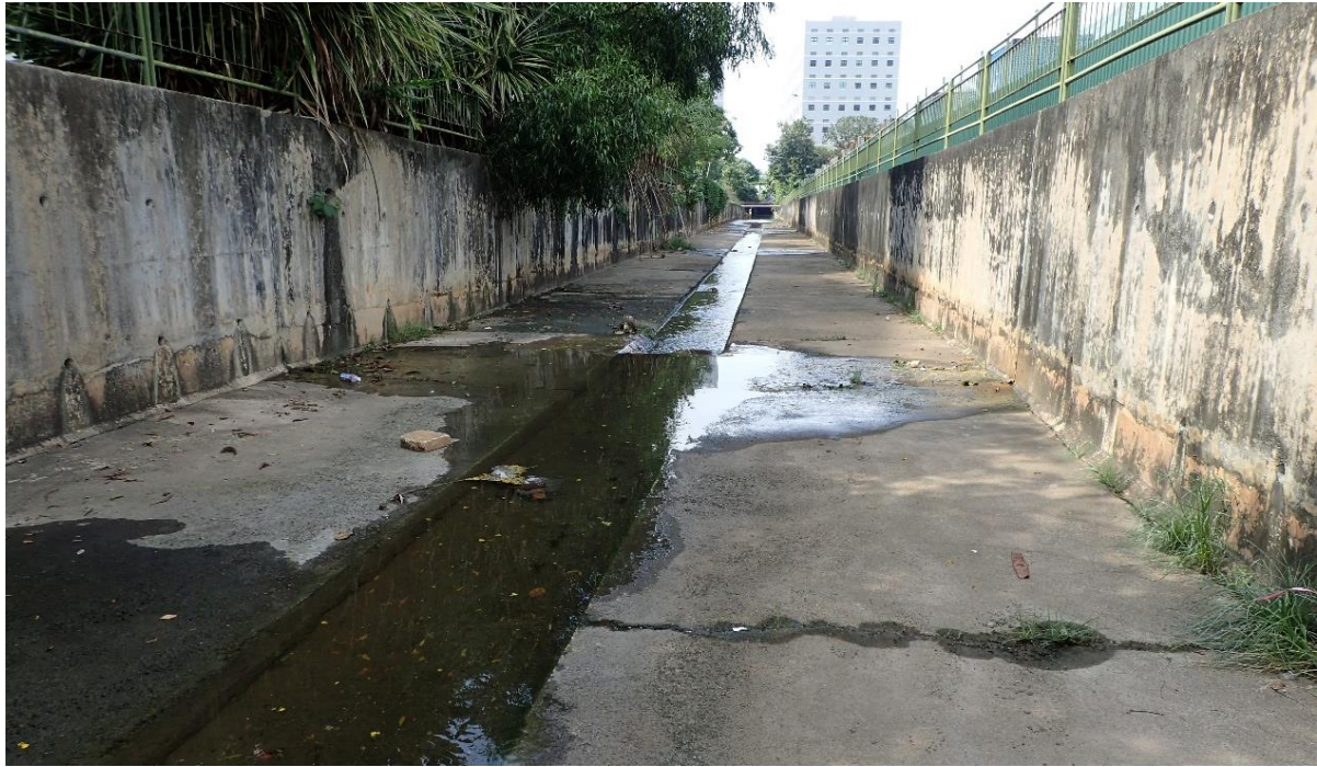
Fig. 1. Section of the concretised storm drain where tarpon leptocephali were obtained on 13 November 2015.
