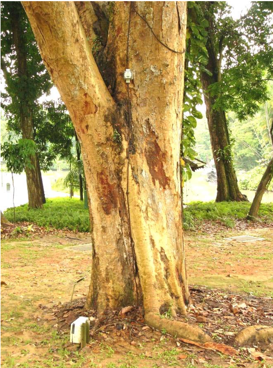
Fig. 24. Lightning arrestor system on a tree in the Singapore Botanic Gardens. Note the cable going vertically up the trunk and the white junction boxes. However, trees in more isolated areas may have their cabling stolen by metal thieves, as has happened in the last few years in Singapore. (Photograph by: Hugh T. W. Tan).
