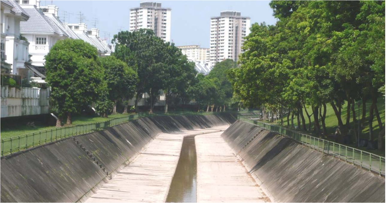
Fig. 6. Sungei Ulu Pandan (“Pandan Canal”) is typical of the canals in Singapore with a low-flow channel in the centre, widening significantly above for high volume and flow rates during downpours. The canals are designed to move water out to the sea quickly, to prevent flooding. However, this makes it difficult to plant anything along the banks, because the fast flows will tear the plants out. (Photograph by: Hugh T. W. Tan).
